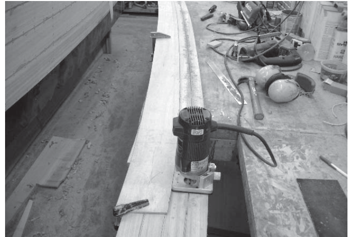
Hold router tight to the stop!
