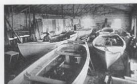
Motor boats under construction.
