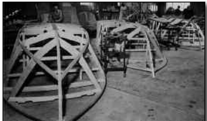
Pre-assembling frames
